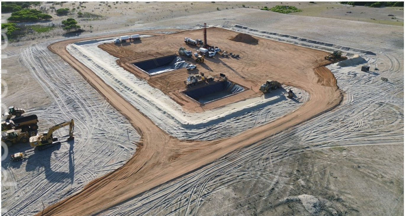
Figure 1: Becos-1 well pad nears completion
