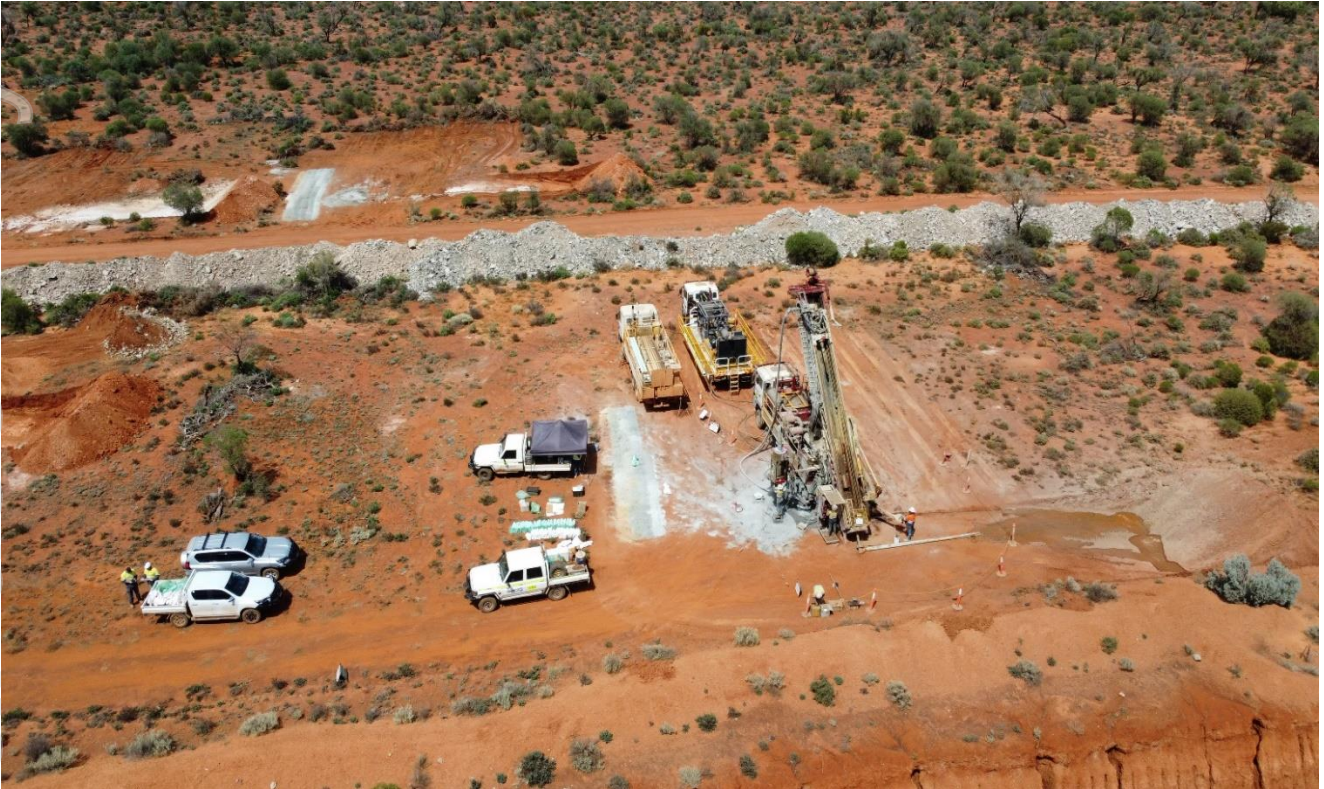
Figure 2 – Photo showing the RC Drill rig on the western side of the Coogee Pit Wall
