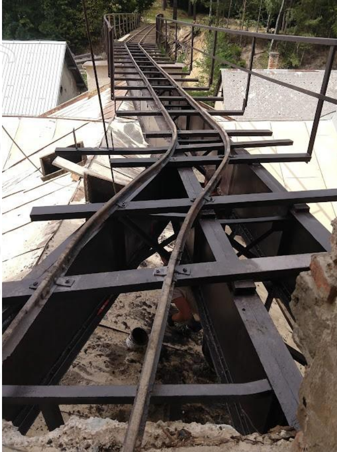
Image 1 (top left): Repair work on the engine room at the Sturec project; Image 2 (top right): Repair work on the engine room at the Sturec project; Image 3 (middle left): cleaning and painting the rail link bridge over the engine room; Image 4 (middle right): near complete roof repairs and installation on the engine room at the Sturec project; Image 5 (bottom left): repair work on the underside of the rail link bridge over the engine room; Image 6 (bottom right): cleaning and painting the rail link bridge over the engine room
