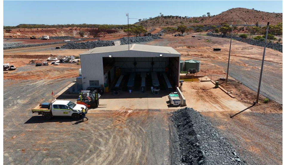
Figure 15 - Sand King – on site core processing facility
