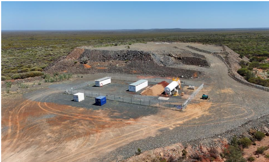
Figure 16 - Explosive and emulsion magazine
