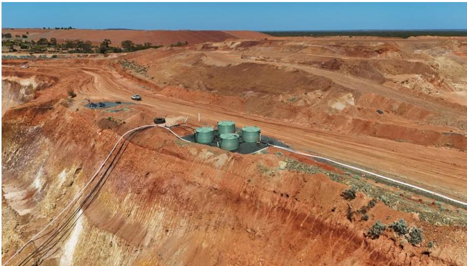
Figure 12 - Sand King header tanks for mine water supply
