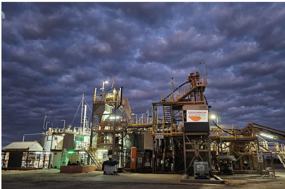
Georgetown Processing Plant
