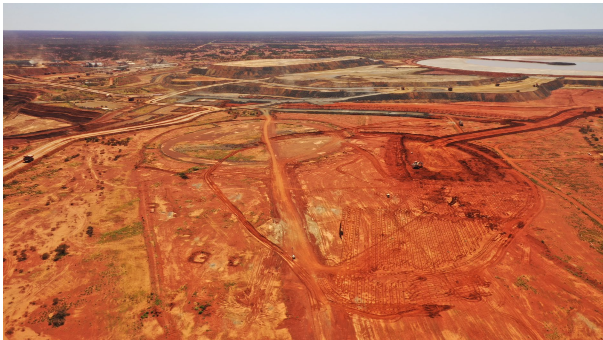
Karlawinda Gold Project – Southern Corridor pre stripping activities
