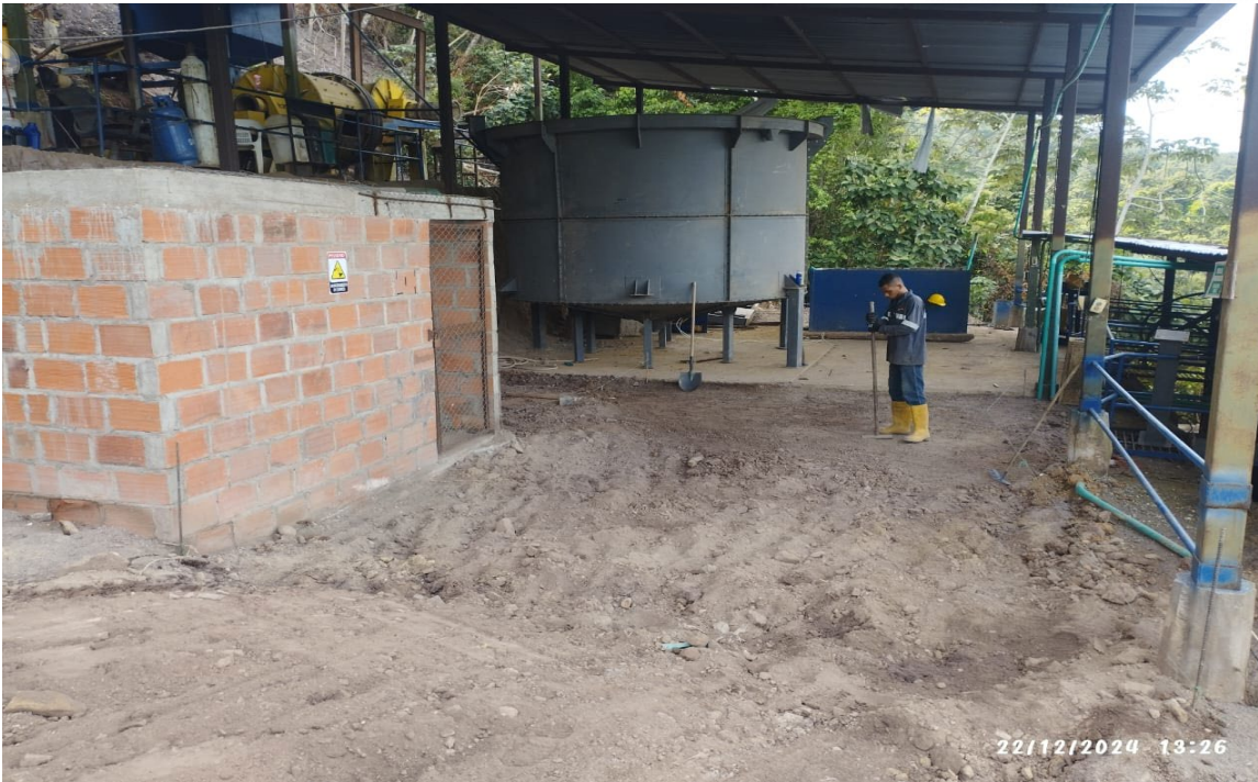
PHOTO 5: NEW THICKENER BEING INSTALLED – SANTA BARBARA PROCESSING PLANT
