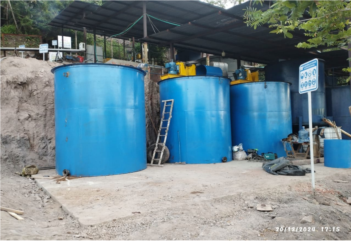
PHOTO 4: NEW AGITATOR TANKS BEING INSTALLED – SANTA BARBARA PROCESSING PLANT
