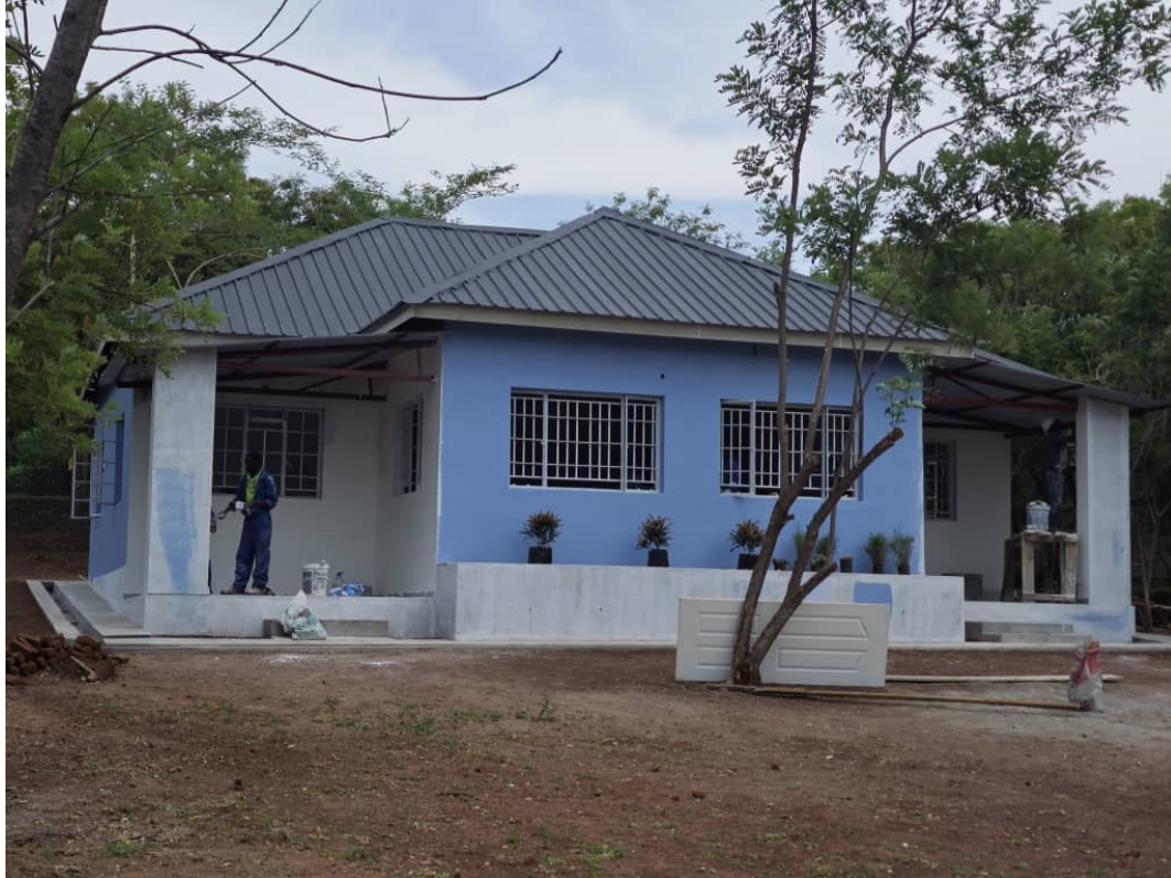
Picture 1: Kangankunde renovated site administration office
