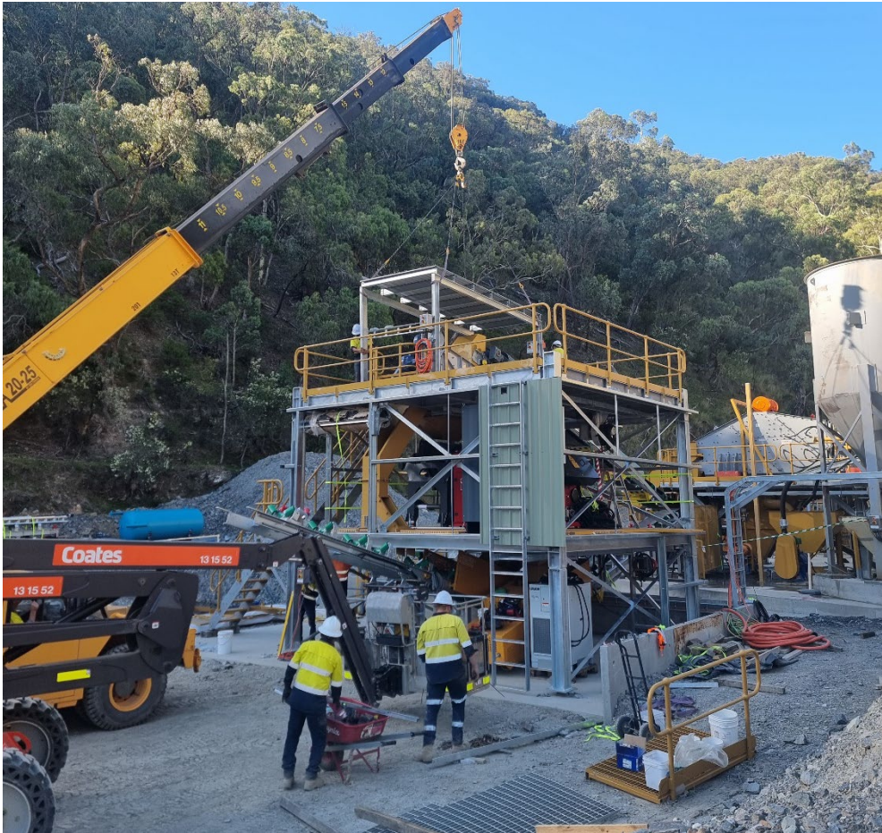
Figure 9 Ore sorter installation well underway
