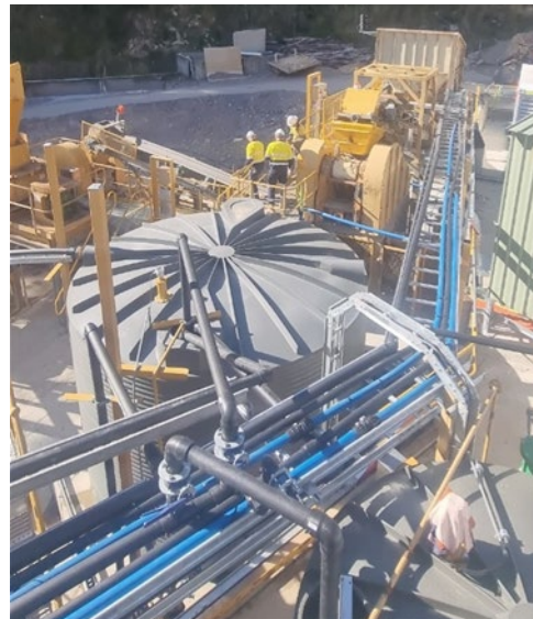
Figure 8 Commissioning team overseeing ore crushing
