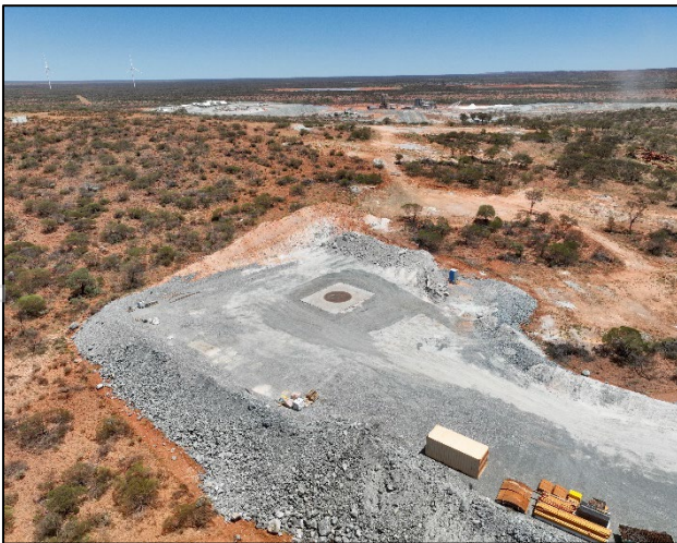
Figure 3: Southern ventilation raise bore site ready for raiseboring activities
