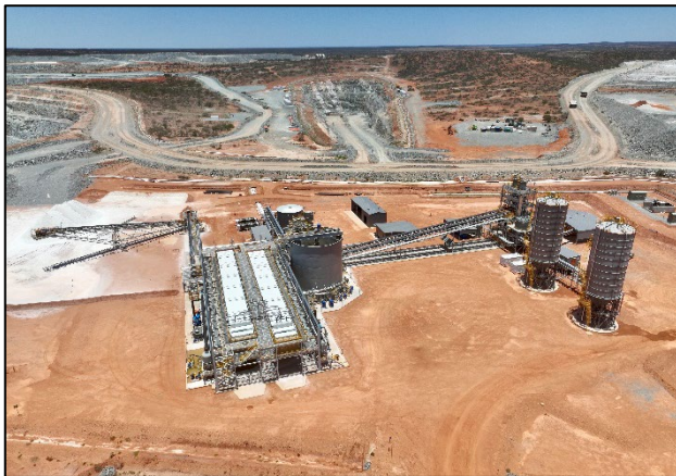
Figure 13: The completed 4Mtpa paste plant
