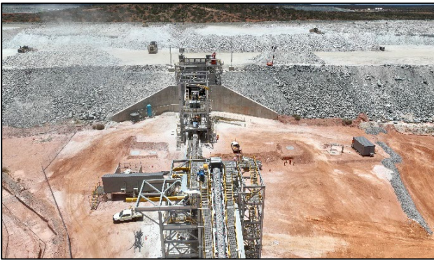
Figure 7: Primary crushing in operation
