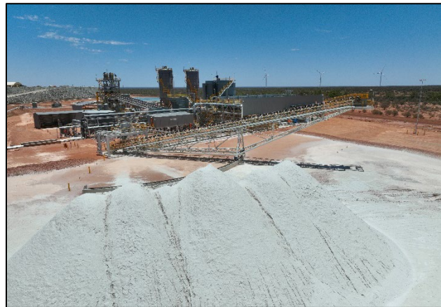
Figure 14: Dry stacking tailings from the paste plant
