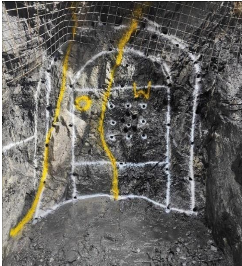
Photo 3. Montezuma exploration drive heading marked-up and ready to be charged
