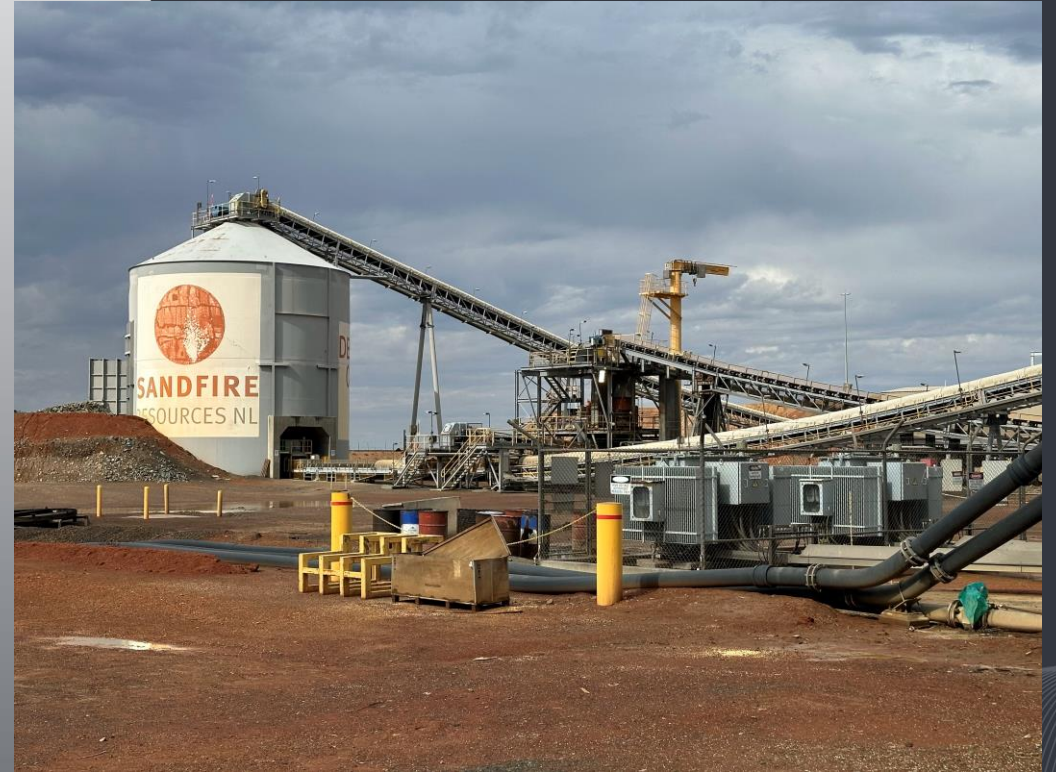
Figure: DeGrussa Process Plant
