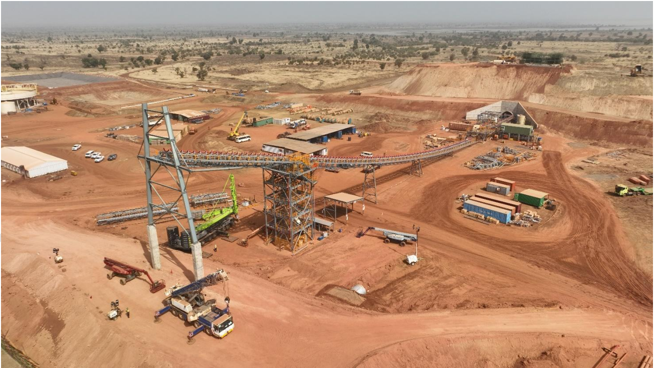
Kiaka Primary Crusher Area
