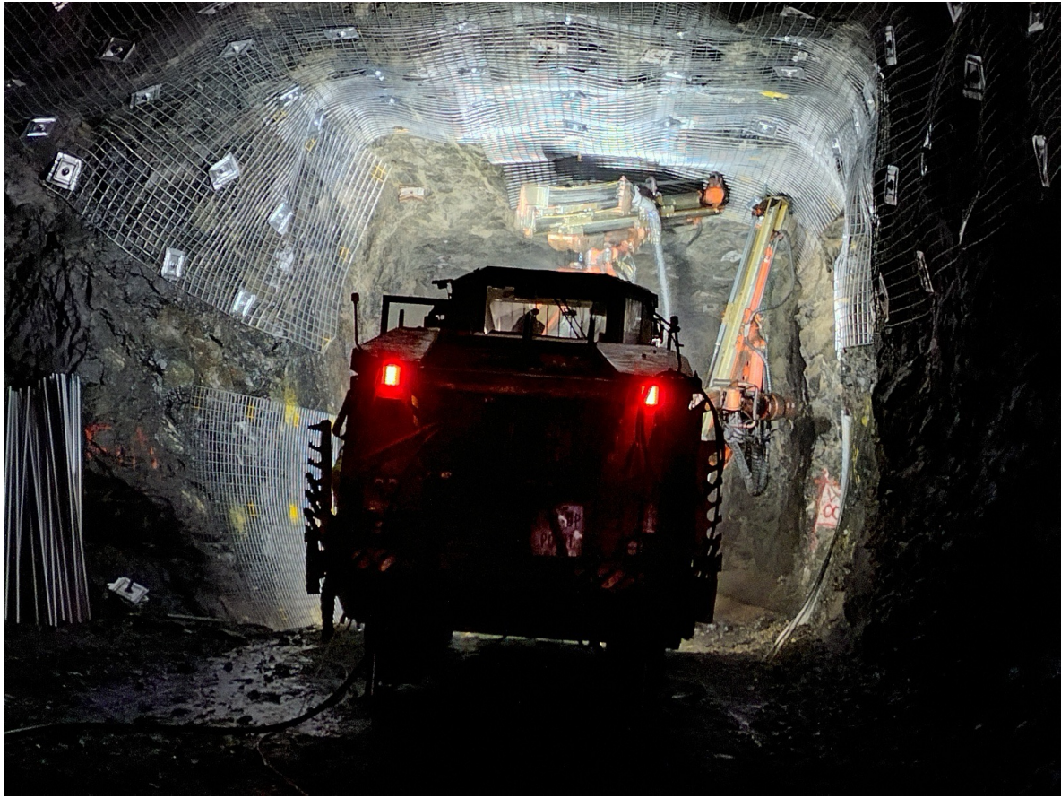
Picture – Rehabilitation of the Bullen Decline underway.
