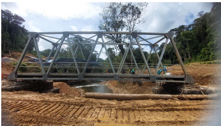
Mohing Bridge development
