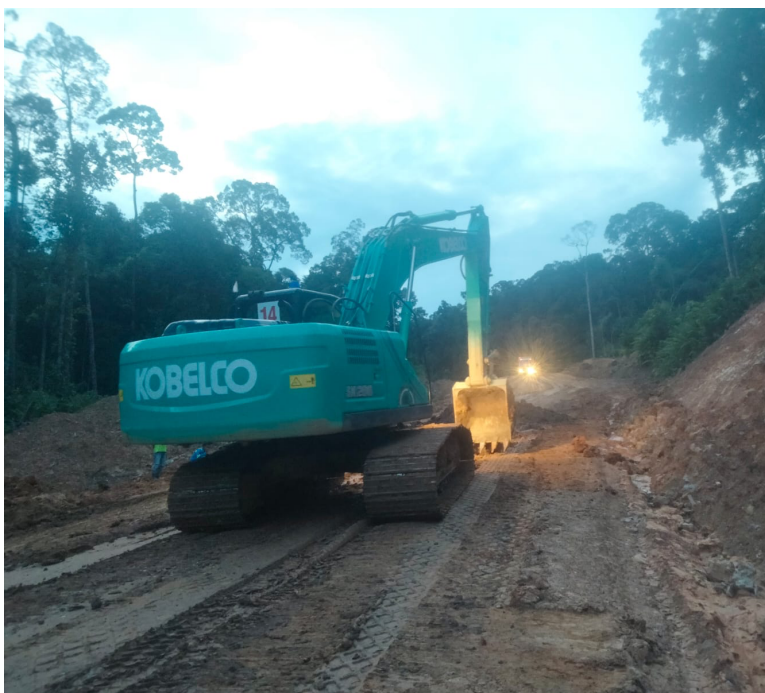
Haul road development
