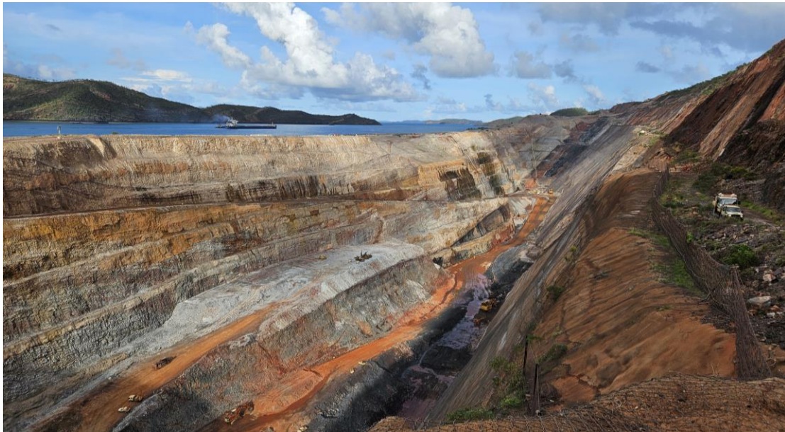
Figure 2: Koolan Island Main pit, eastern half, showing ongoing excavation of the former eastern mine haul ramp (centre) and high grade iron ore mining along the footwall (right hand side), as a loaded bulk ore vessel departs, January 2025.
