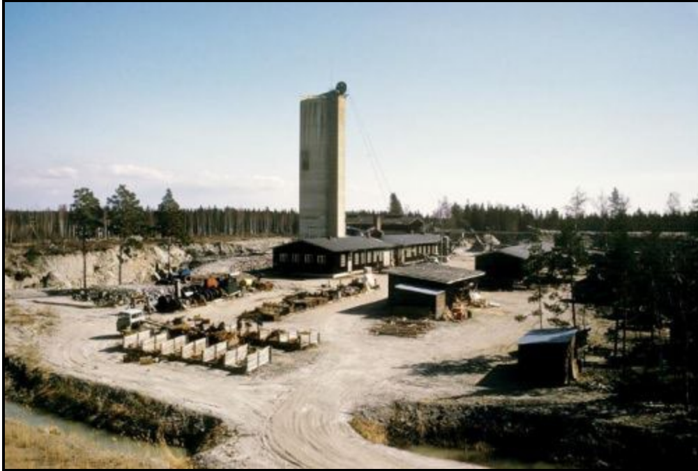
Korsnäs Minesite laydown area in 1970 - location of current core processing facilities.
