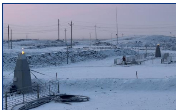
New pilot wells with initial gas flares
