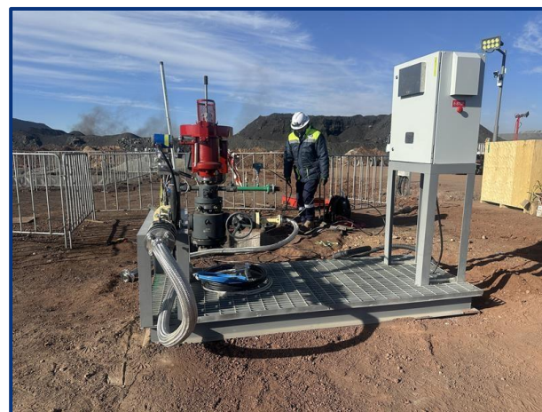
Completion and final commissioning of the additional Lucky Fox pilot wells
