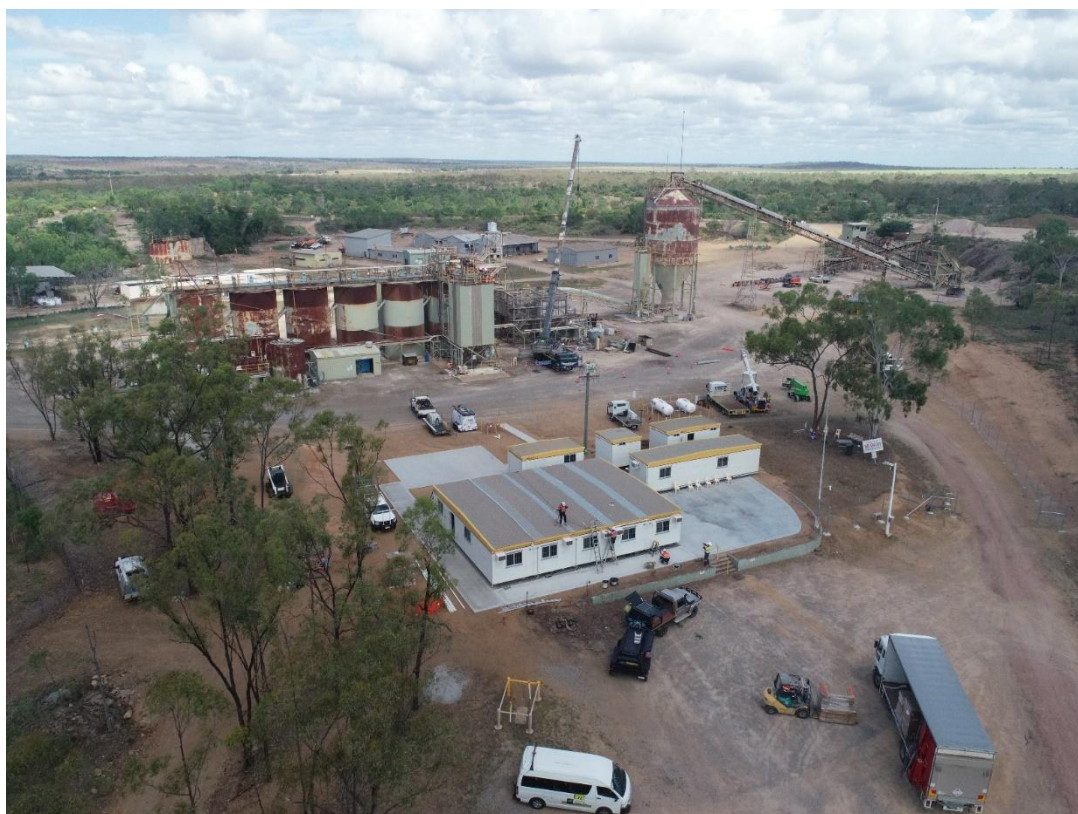
Figure 1: Construction at the Blackjack Gold Processing Plant near Charters Towers, QLD.
