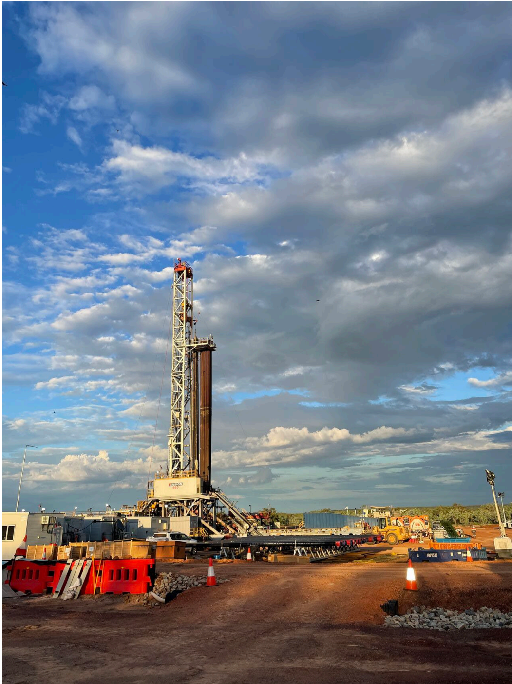
Carpentaria C5 Ensign drill rig on location in EP187
