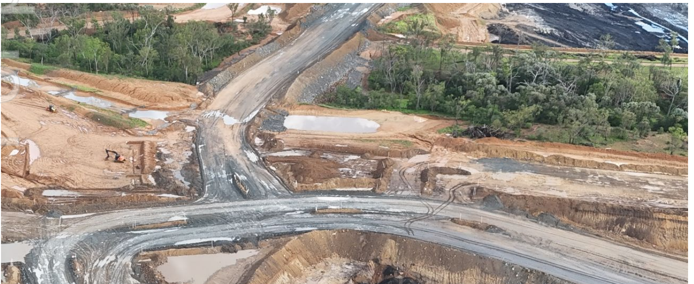
Figure 2: Teviot Creek Crossing Construction (looking North)
