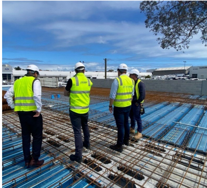
Figure 6: Inspection of installed works – Audi Myaree Project
