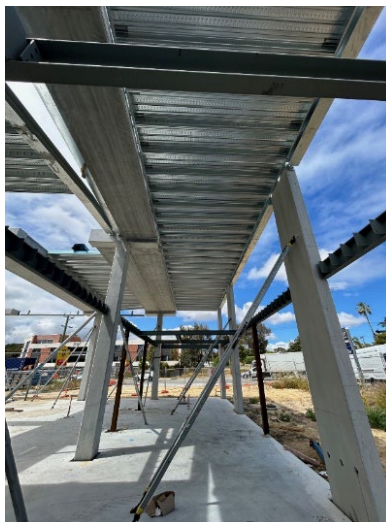
Figure 2: Installed SlimDek
