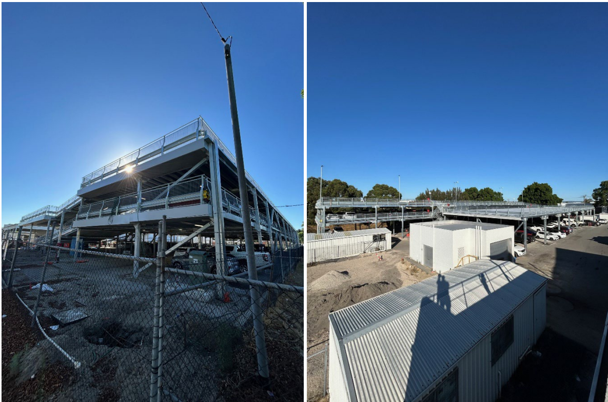
Figure 4 & 5: Substantial completion at Forward St
