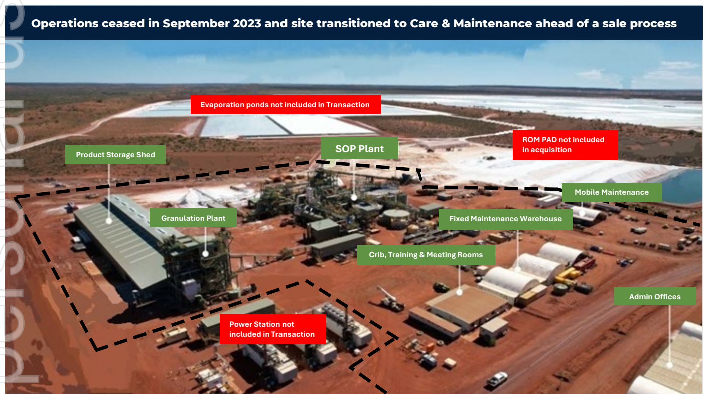
Figure 1 – Photograph of the Beyondie Potash Project in 2023 when in operation by Kalium. The Transaction comprises a fully constructed processing plant, site offices and maintenance infrastructure. Specific plant components include, KTMS crushing circuit, Kainite conversion circuit, column flotation circuit, liquor cooling heat exchangers, evaporative cooling circuit, product separation centrifuges, SOP recovery and granulation unit, RO water plant and a bulk storage shed.
