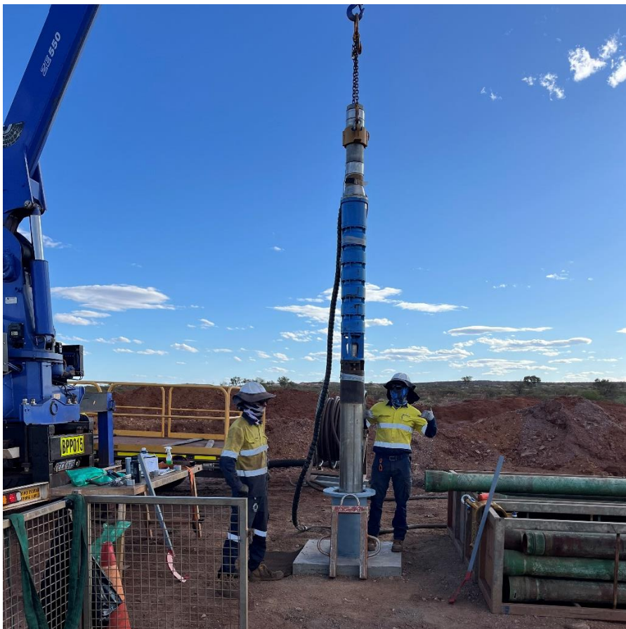
Installation of high flow test pump at Woodie Woodie
