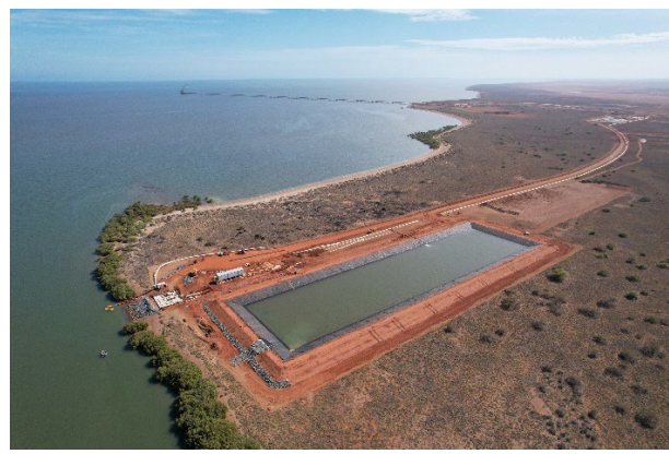
Figure 4: Construction of the secondary seawater intake station
