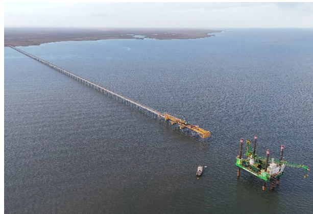
Figure 2: Jack-up barge arrives at Mardie to install the jetty head
