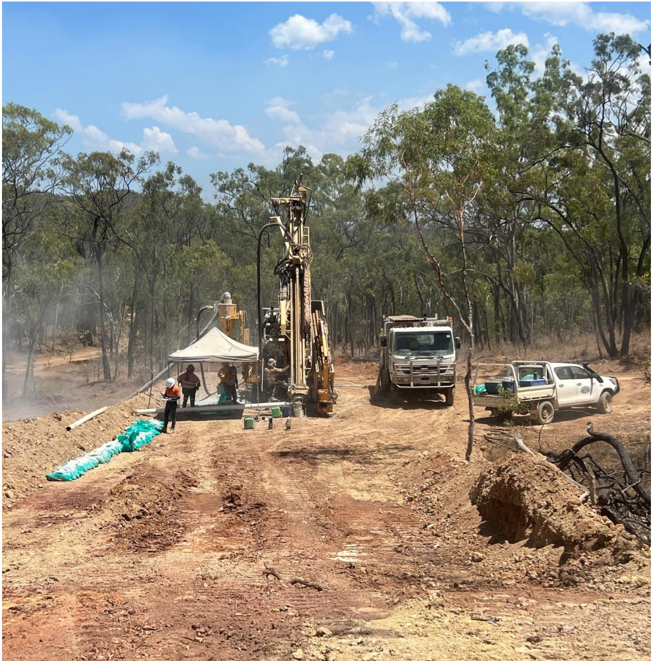
Figure 1 Orient East Drilling (October 2024)
