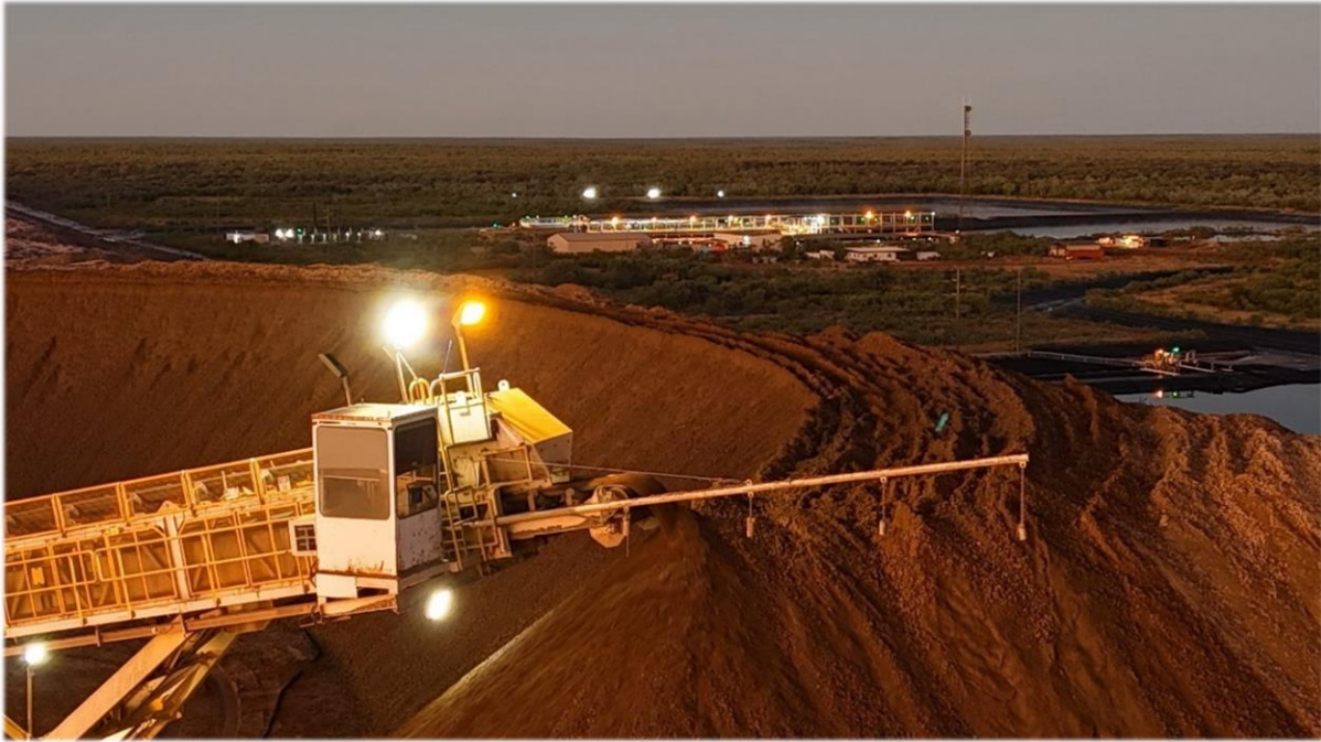
Figure 5: Radial stacker starting pad 21
