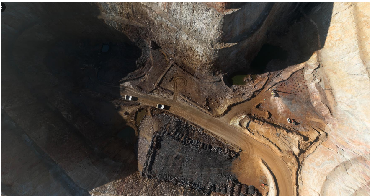
Figure 3: AHW Nearing Completion
