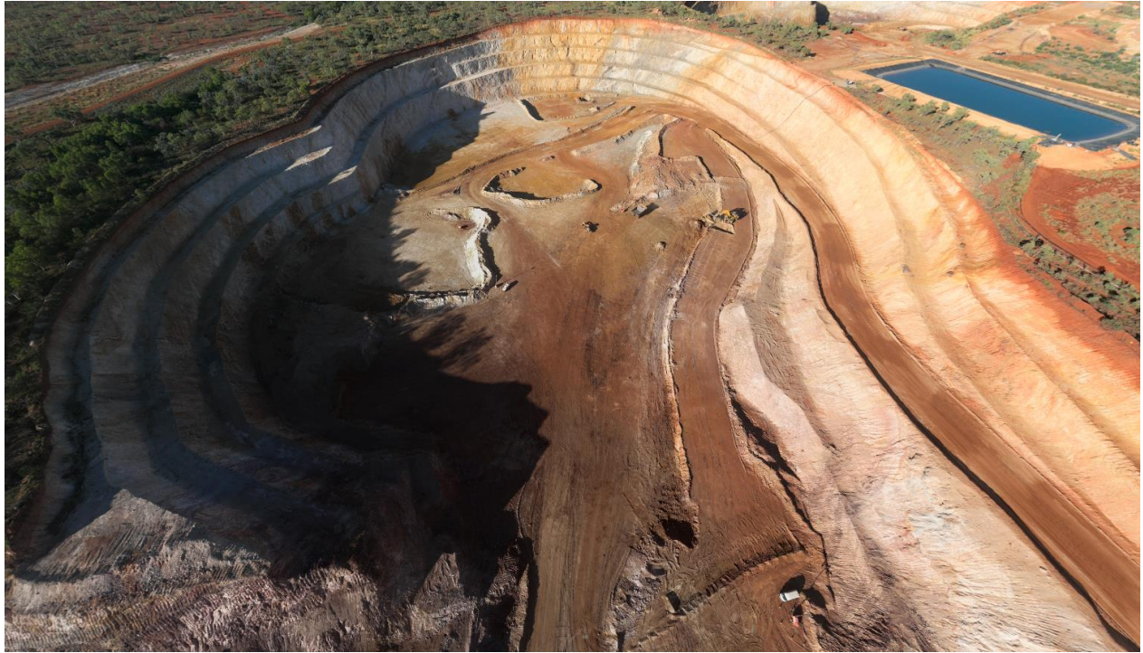
Figure 2: AHE Stage 2 progression through 300 and 295RL benches
