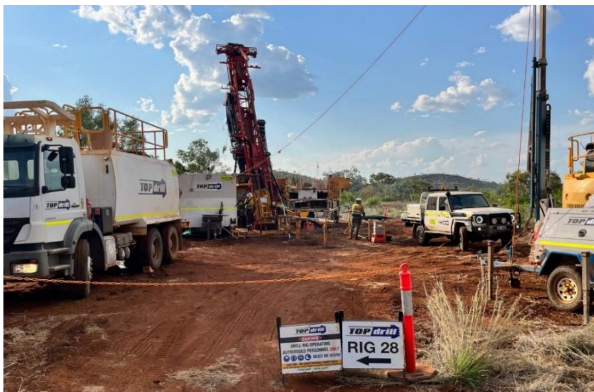
Photo One | Topdrill at the first hole for Eileen Bore drilling
