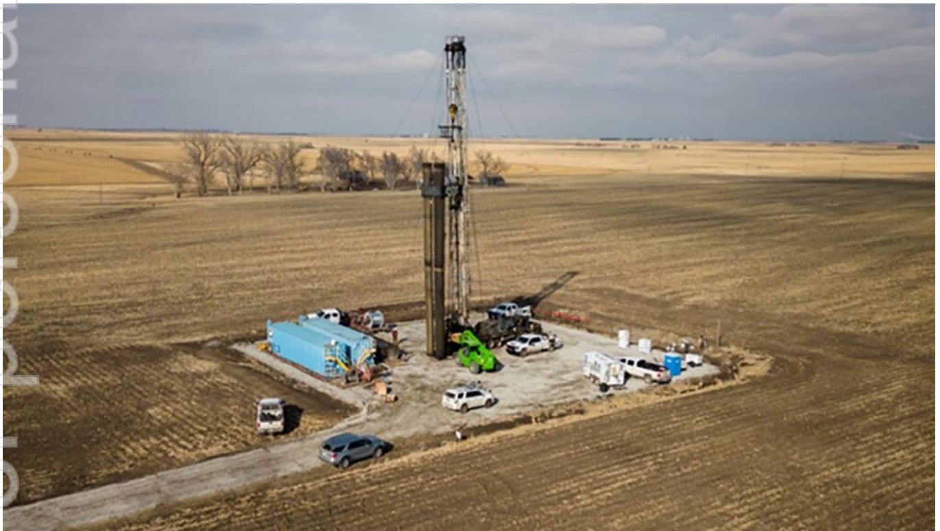
Figure 4. Wildcat well specifically targeting white hydrogen (Hoarty NE3) in Geneva, Nebraska.
