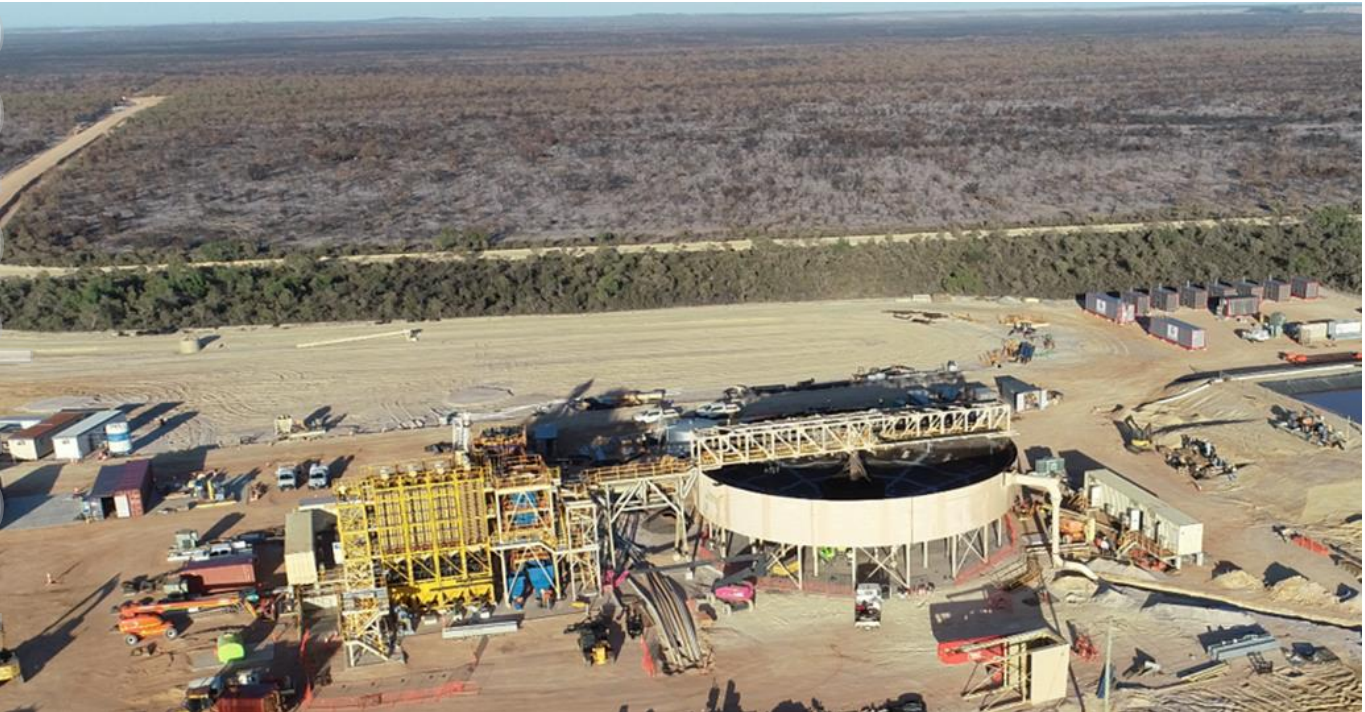
Figure 2: WCP (Flex Plant) & Thickener Construction
