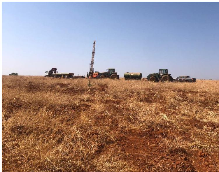
Figure 5: Enova's CODA North Tenements: Vast pastureland with REE mineralisation potential (Enova's Contract Diamond Drill Rig working on the horizon)
