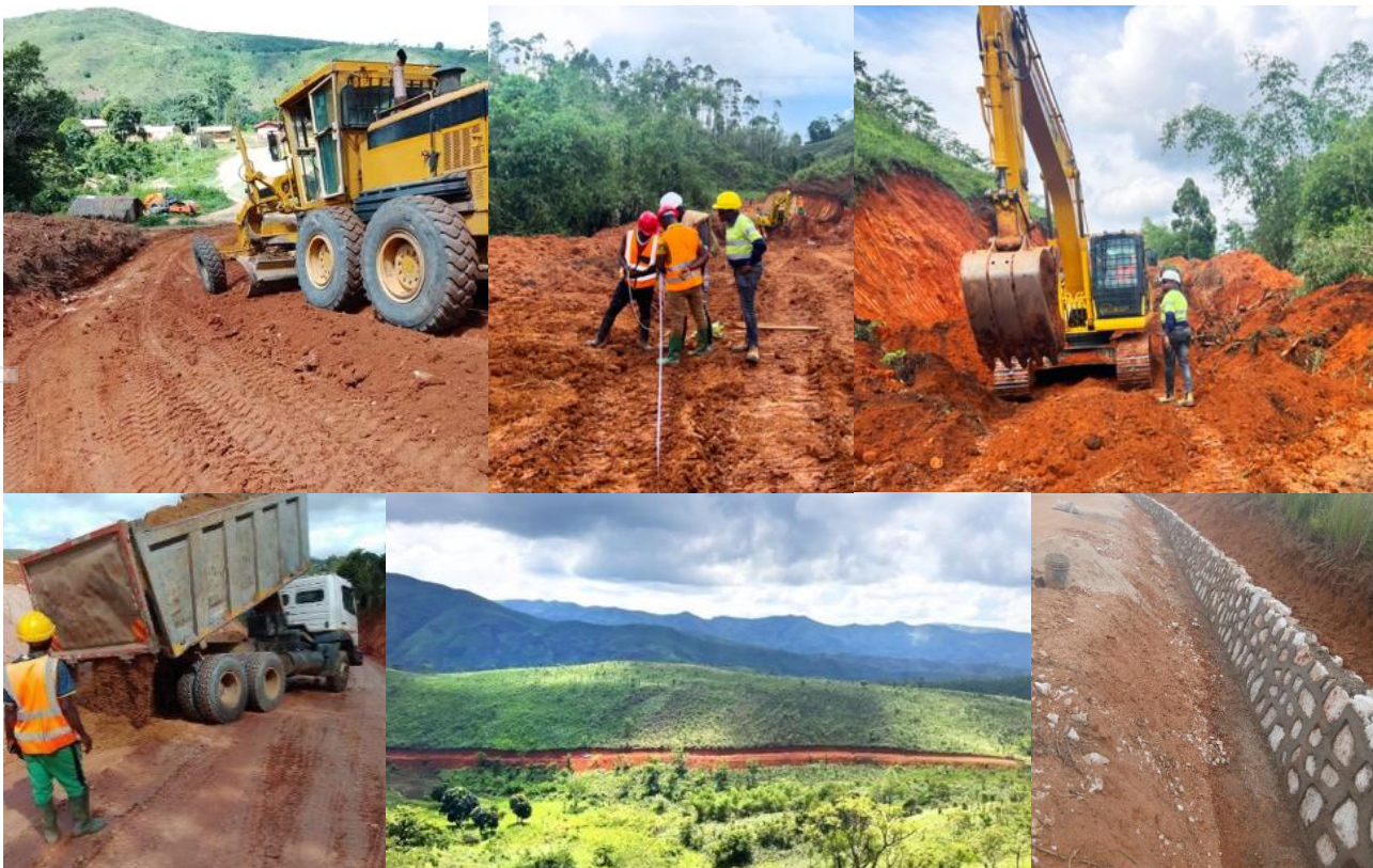
Southern road upgrade
