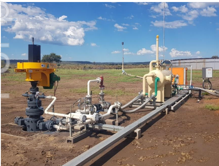
Figure 3: Mahalo East pilot production facilities
