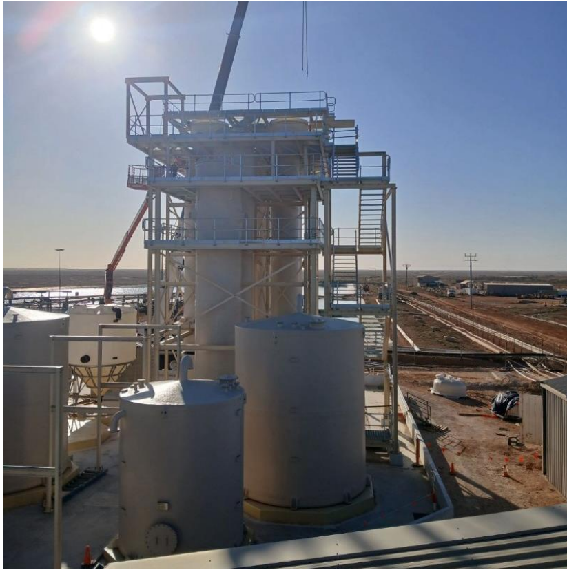
Mechanical installation complete for Heathgate Uranium Processing Plant
