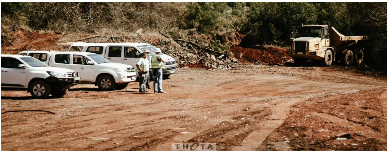
Figure 1: Plant site earthworks preparation for dolomite drilling
