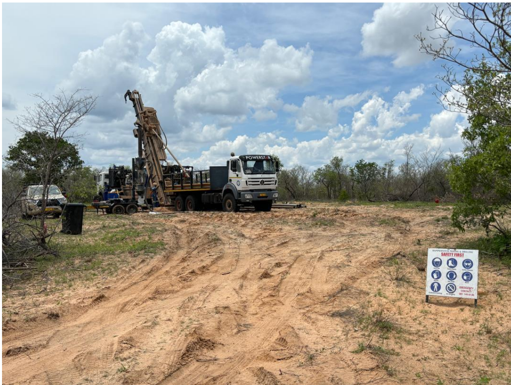
Figure 7: Drill rig mobilising at the Damara Copper Project.
