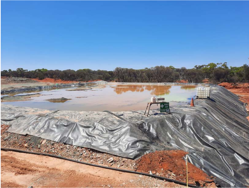
Figure 6: Vat 1 complete and full of ore, water and cyanide, December 2024
