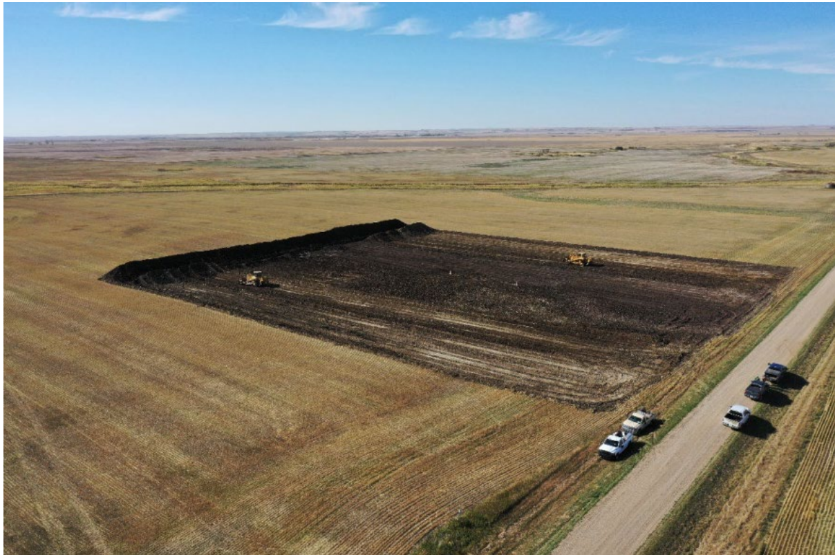
Figure 1: Pad #3 Successfully Cleared
