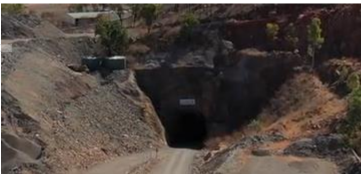
Figure 6. Mungana underground portal (Source: Auctus Resources)
