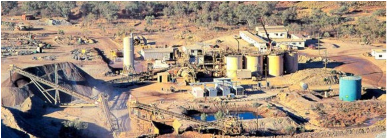
Figure 6: Butchers Creek gold processing plant. Circa 1996
