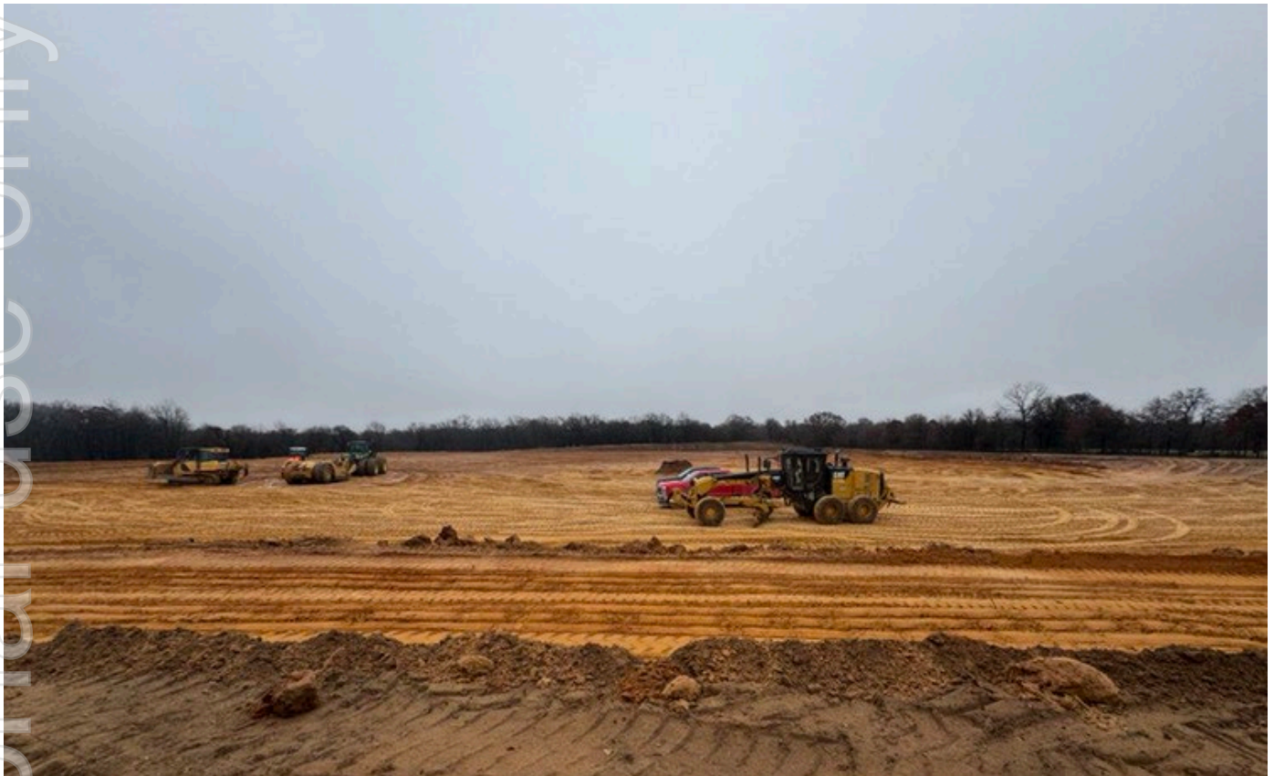
Figure 1. Construction of the Bruins Well all-weather drilling pad.
