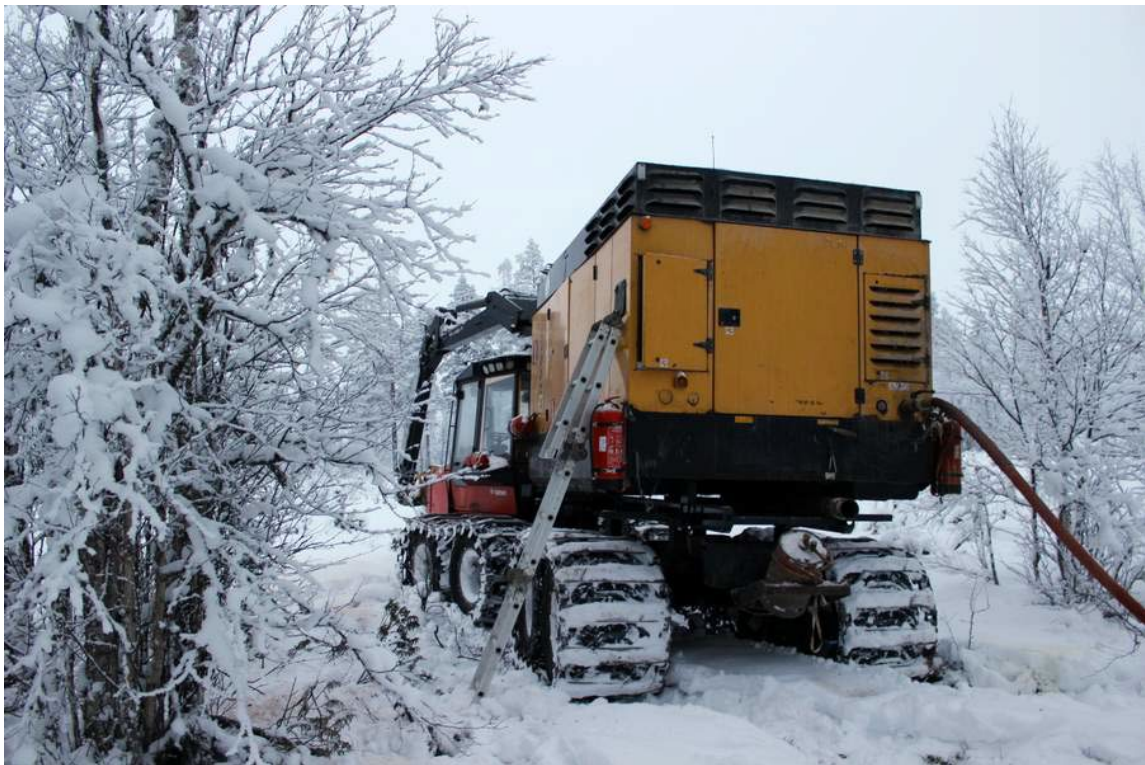
Figure 4: The RC drilling rig that will be mobilised to KSB Project site.
