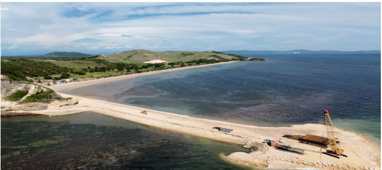
Pictured above: Sheet piling delivered to the CLP project site.
