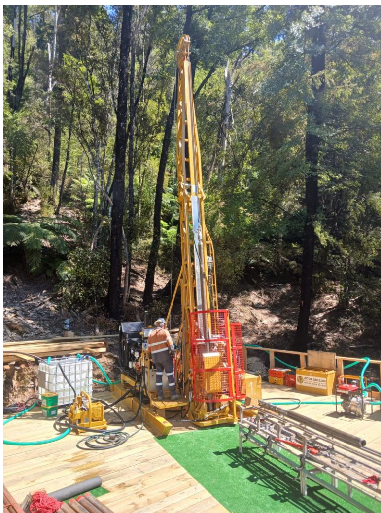
Figure 7. Diamond Drilling rig commences new deep hole at Sams Creek.
