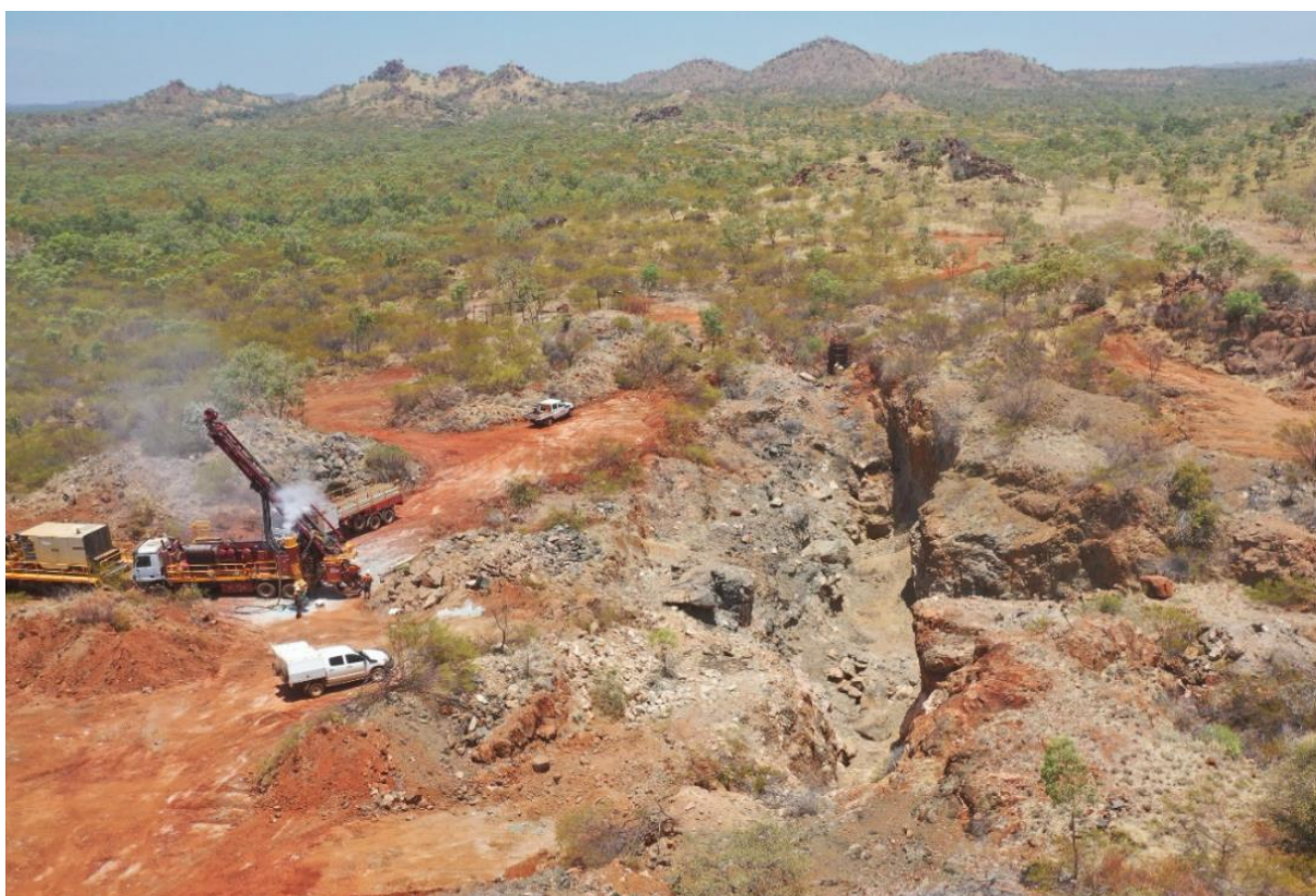
Figure 2: Photograph of the drill rig during the first phase of drilling at the Surprise Copper Project
