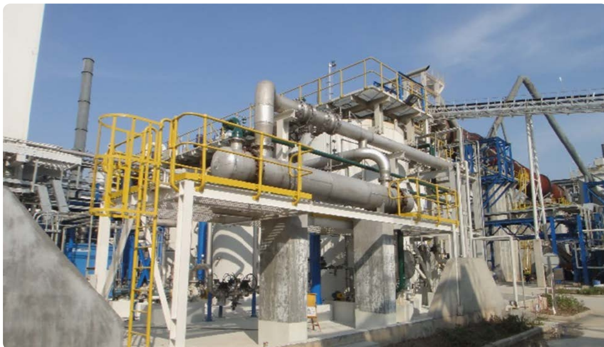
Figure 2C: Galaxy Jiangsu Lithium Carbonate Plant
