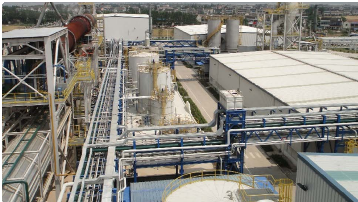
Figure 2B: Galaxy Jiangsu Lithium Carbonate Plant
