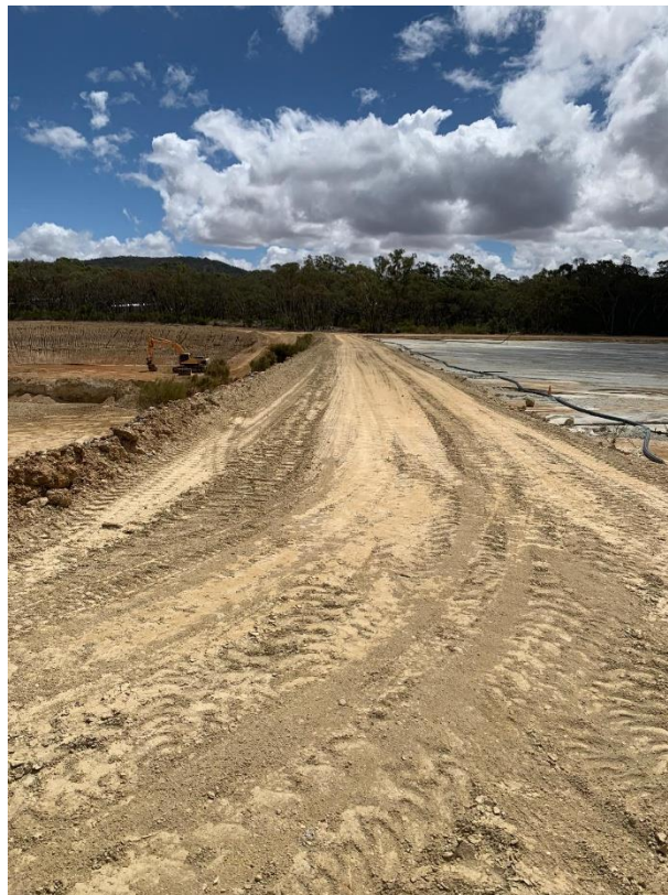
Figure 6: Looking west across the western portion of the TSF5 D lift
