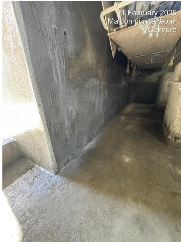
Figure 7: Photo of a section of the replacement high strength concrete foundation of the processing plant, that supports the ball mill.
