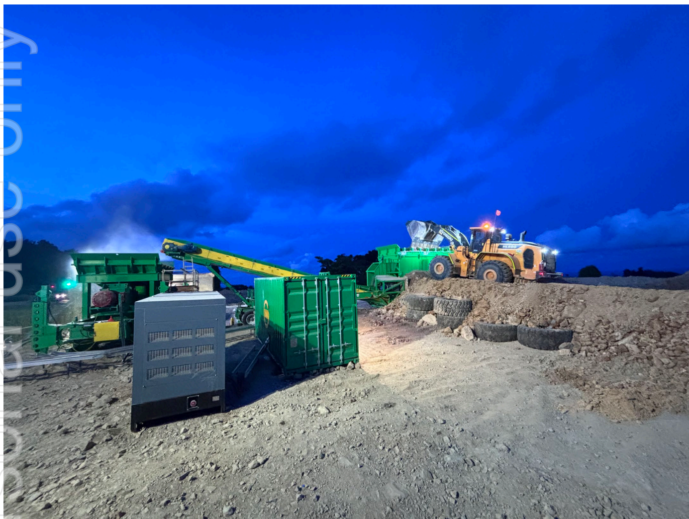
Figure 2. MMD Sizer Commissioning at Sorowar ROM Pad
