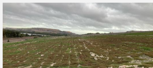
Peak Downs Rehabilitation Works
