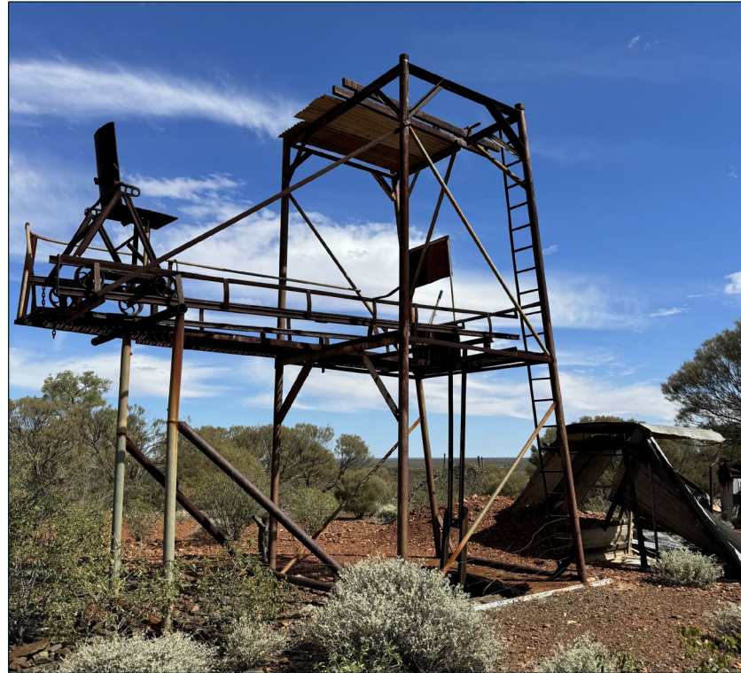
Barrambie Range North Shaft c.1970's
